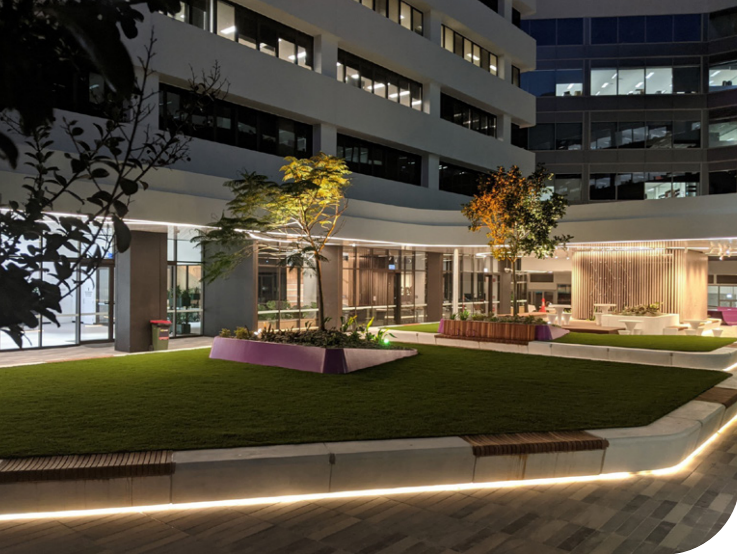
100 Wickham Street Fortitude Valley Brisbane, Queensland
